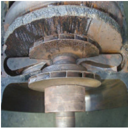
Once the bundle was removed from the case, the outside of the return channels broke clean away from the diaphragms.
