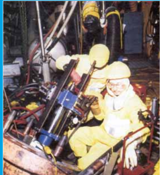
MSIV repair in containment at Nuclear Plant
