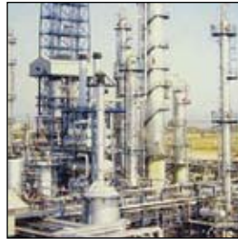
Worldwide maintenance and repair in oil refineries
