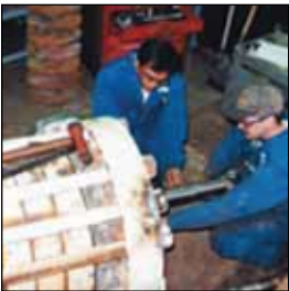
On site repairs by expert personnel
