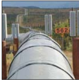
Provision of oil pipeline maintenance
