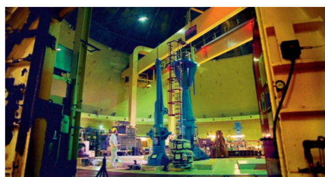
Goliath crane at United Kingdom Atomic Energy Authority Dounreay plant in Scotland, UK
