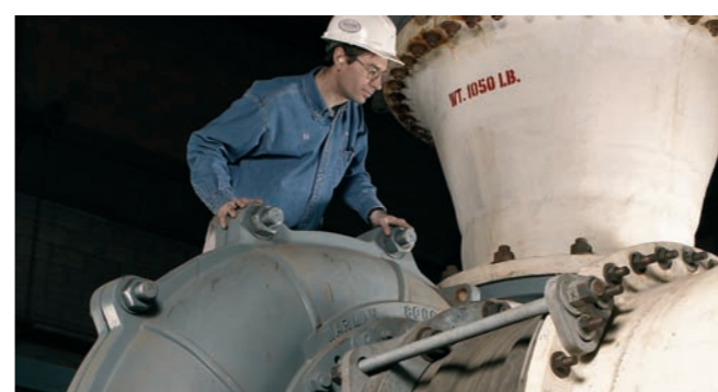
Warman type GSL centrifugal slurry pump on FGD absorber recycle duty in the USA
