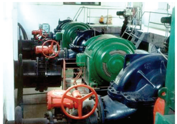
Photos: Above, installation of Weir Split Case pumps.
